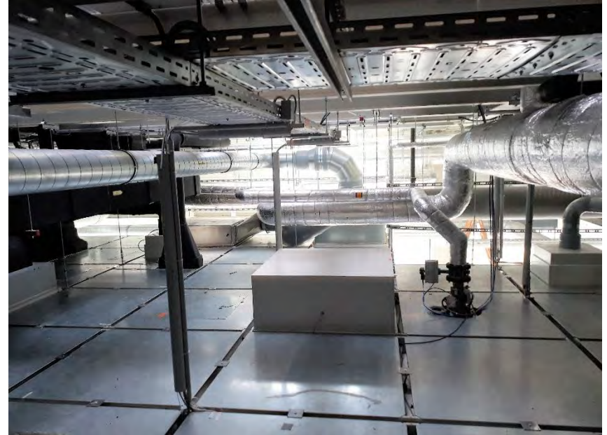
Clean room ceiling, walkable
