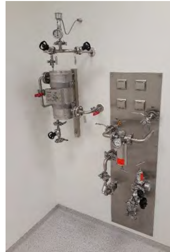
Clean steam sampling and media panel
