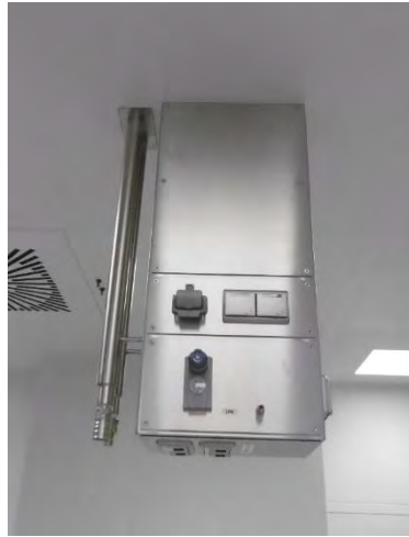
Connect panel from cleanroom ceiling (keeps flexibility on floor)
