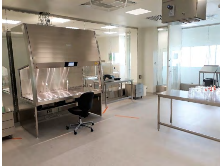
Production area (during installation / IQ)
