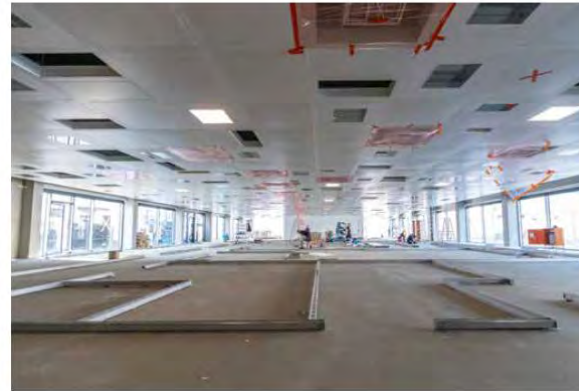
Cleanroom floor installation work
