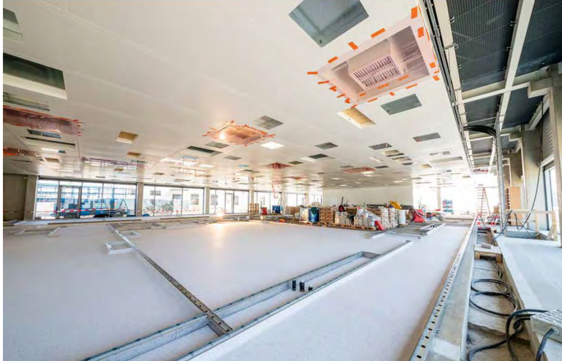
Cleanroom floor installation work
